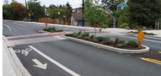
Example of a unsignalized midblock crossing
