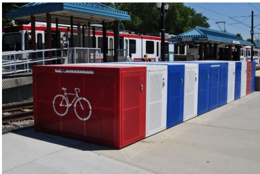
Example of bicycle lockers
