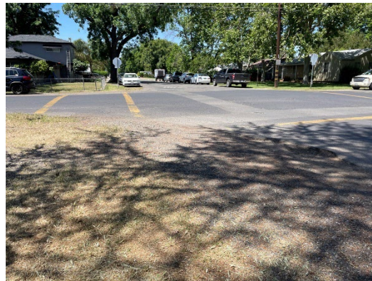
Arbutus Avenue and East 3 rd Street pavement and crossing conditions
