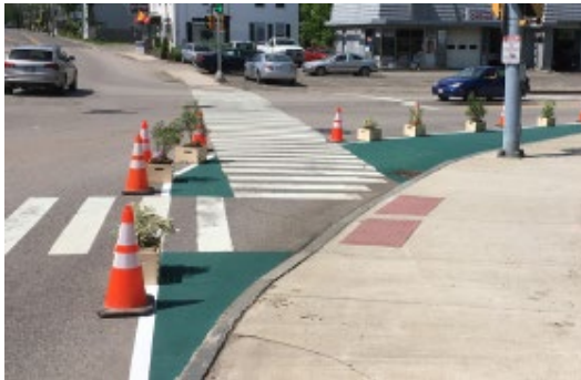
Curb extension in Portsmouth, NH using colorful surface treatments, cones, and plants
