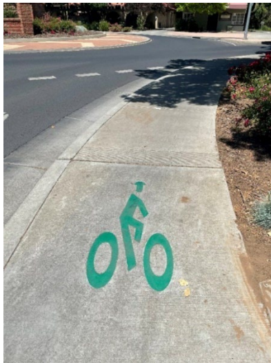
Green in-pavement markings indicating the presence of bicyclists on sidewalks approaching a roundabout in Chico
