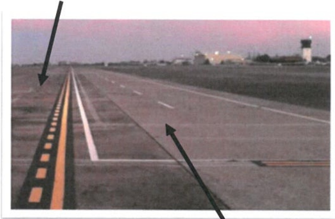
Vehicle Travel Lane (non-movement area side)
