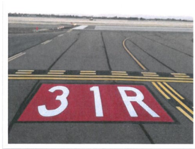
Surface Painted Holding Position Marking
