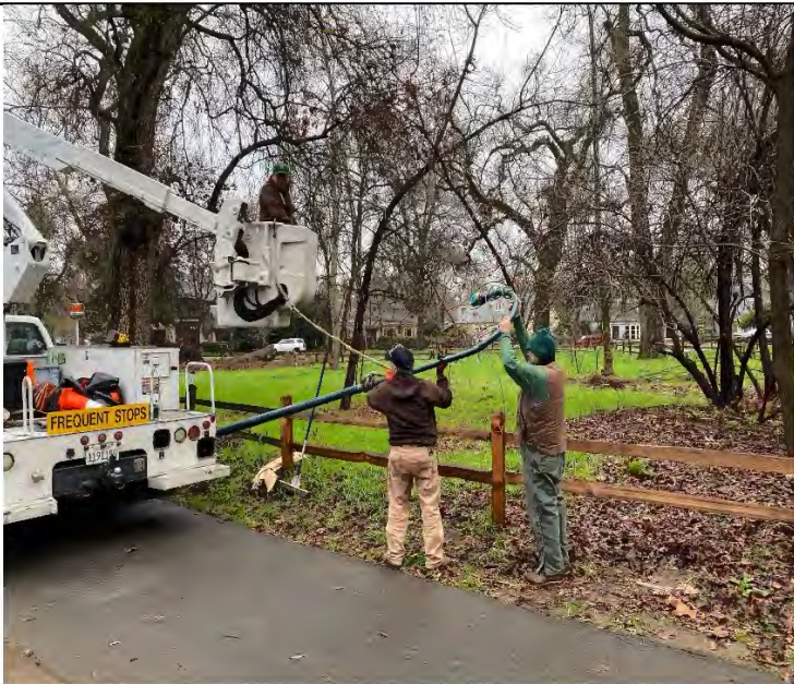
Light Pole Replacement
