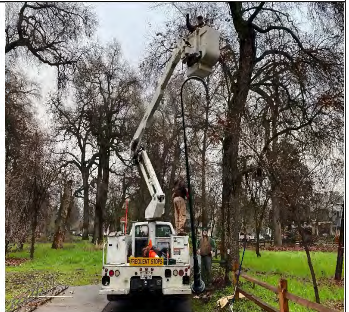
Light Pole Replacement
