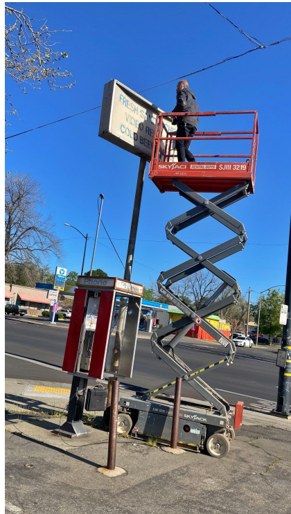
Inspecting/assessing existing sign "can"
