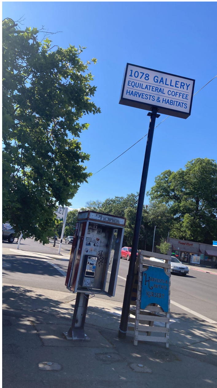
Completed sign installation
