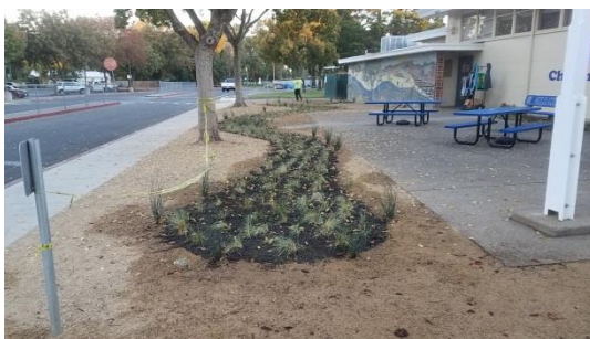
Photograph 2: Chapman Elementary School.
