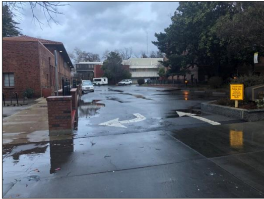
Photograph 1. Flowing water from the church parking lot
